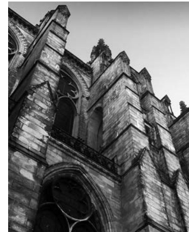
Buttresses at Cathedral of St. John the Divine photo credit: Polly Barton
